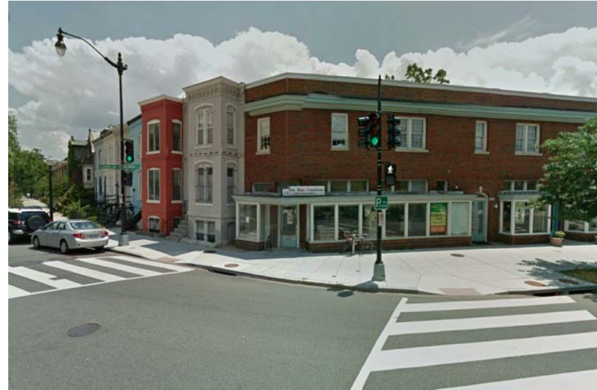
Florida Ave & Champlain Street, Facing SE
