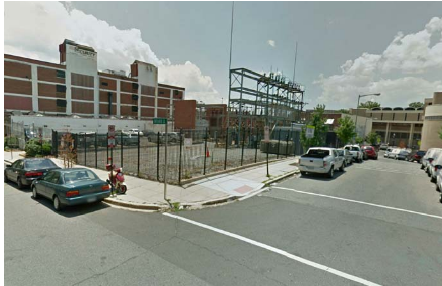
Pepco Facility Along Ontario Rd, Facing SW
