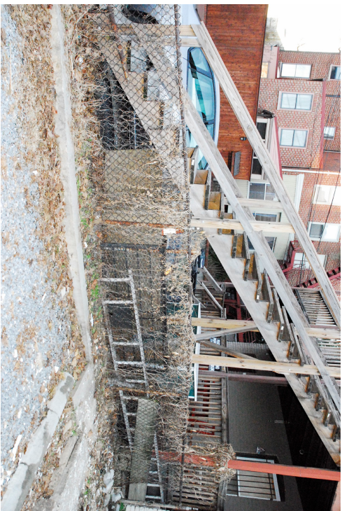
Construction in Rear Yard of Adjacent Structure
