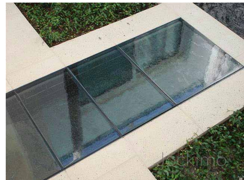
AREAWAY, STRUCTURAL GLASS ROOF
