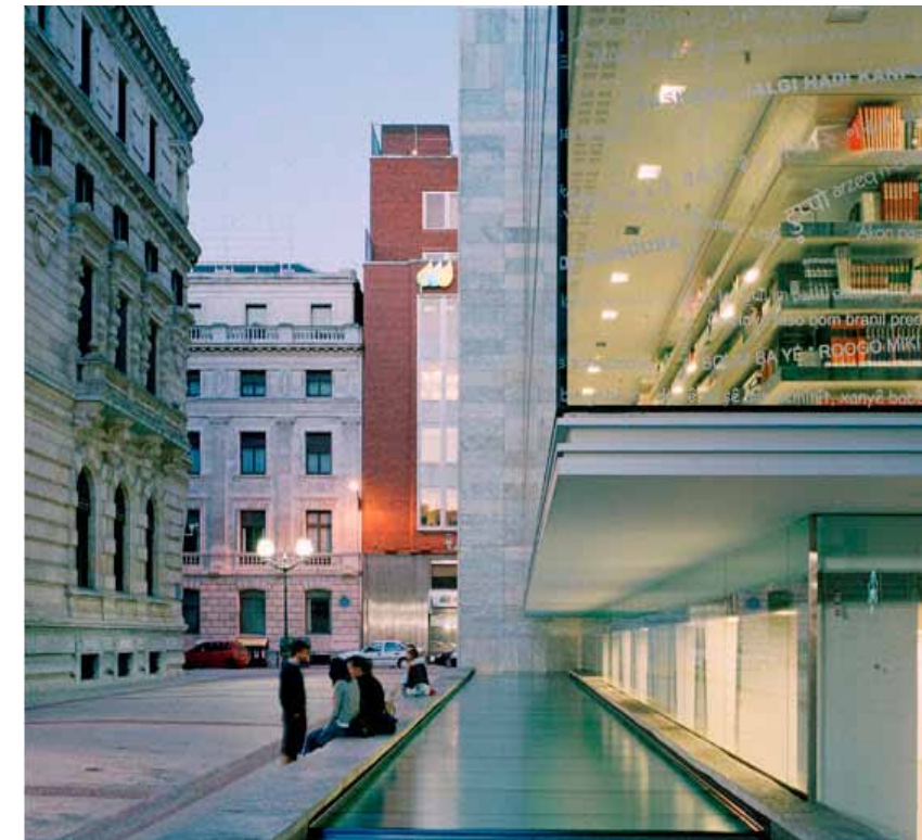
AREAWAY, STRUCTURAL GLASS ROOF
