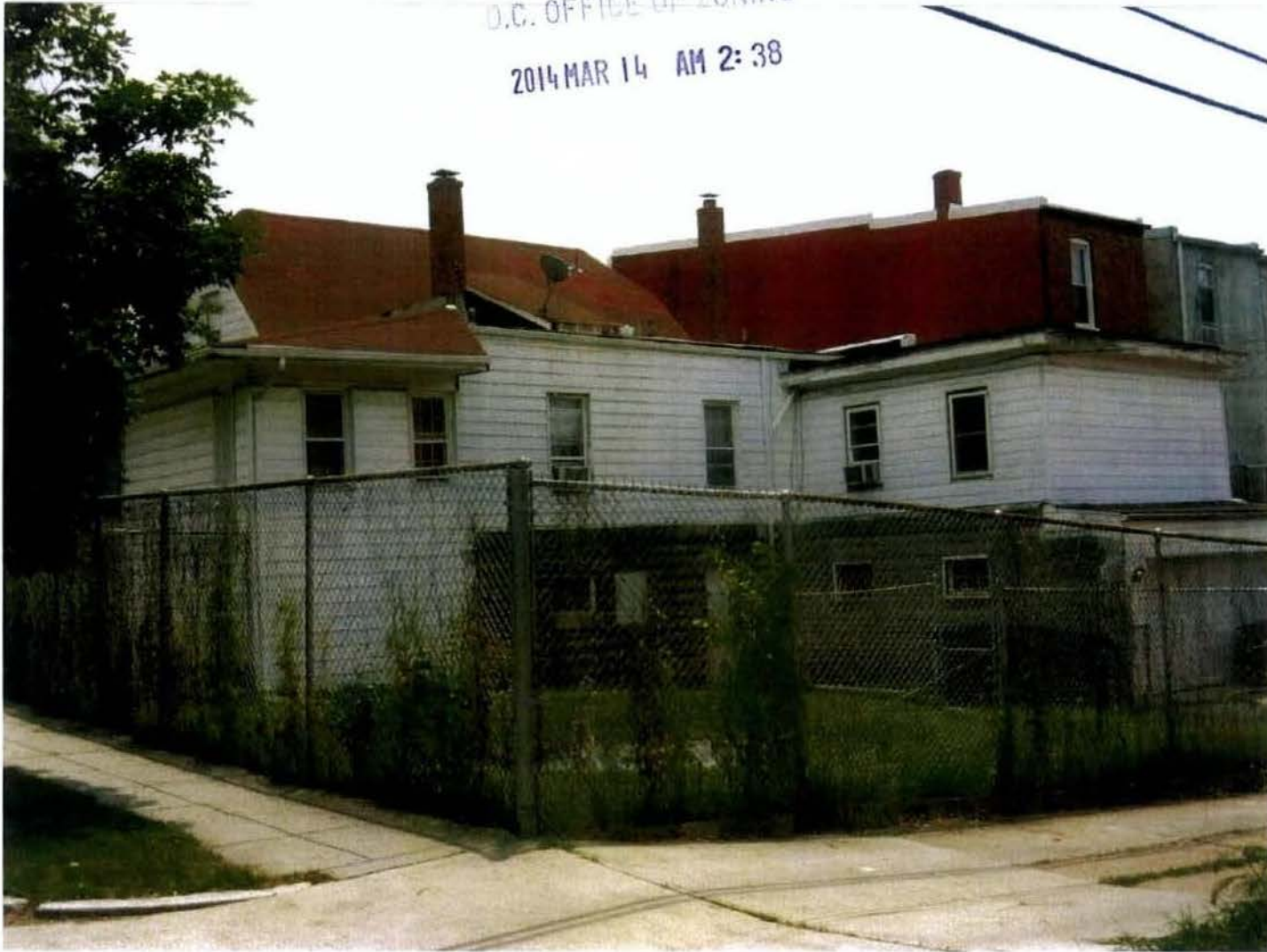
EXISTING CONDITIONS REAR ELEVATION AT ALLEY
