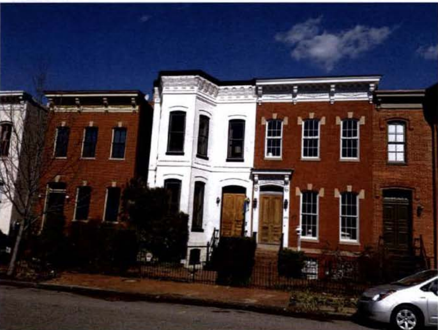
630 A Street SE Street view 3
