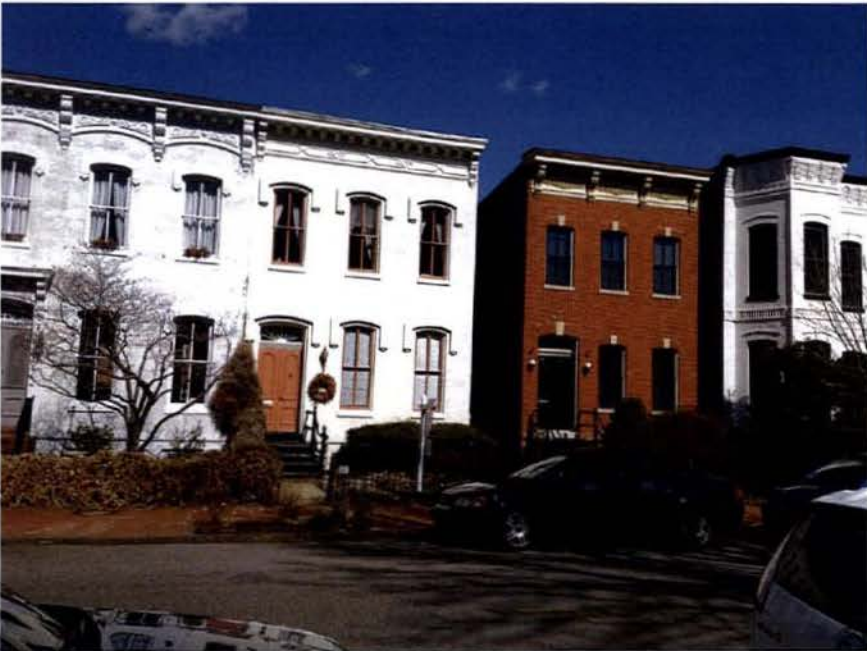
630 A Street SE Street view 2
