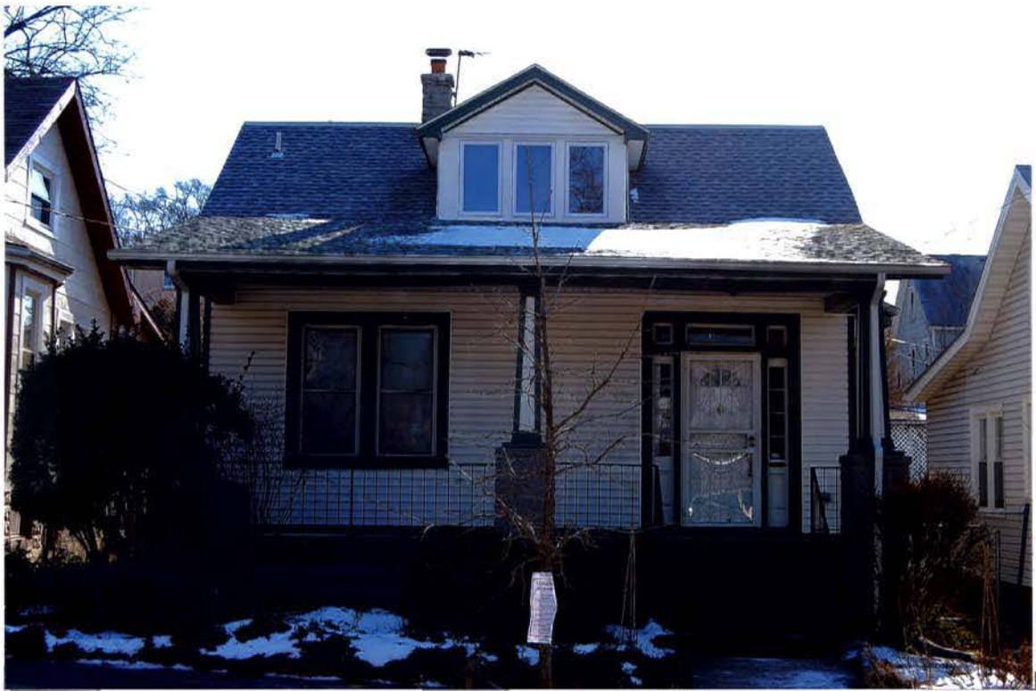
FRONT - 1005 OTIS STREET, N.E.
