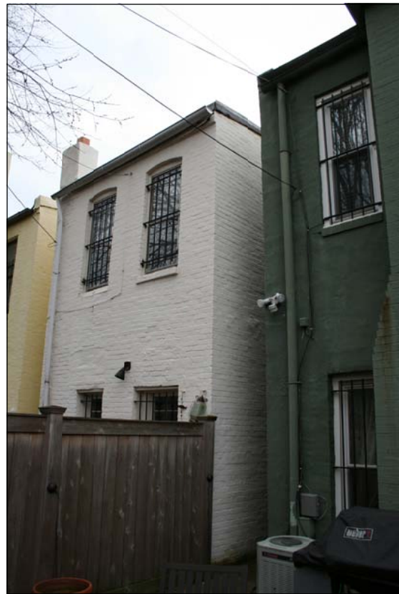
View from rear yard towards Southeast
