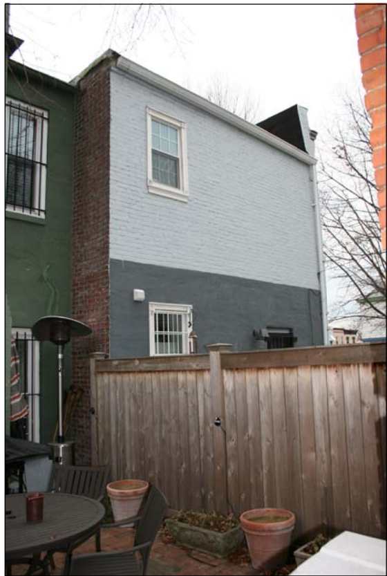
View from rear yard towards southwest
