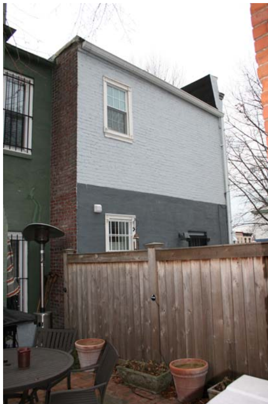
View from rear yard towards 1400 E Street SE
