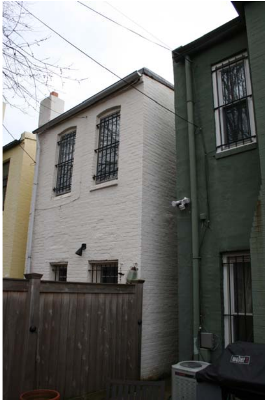
View from rear yard towards 1404 E Street SE
