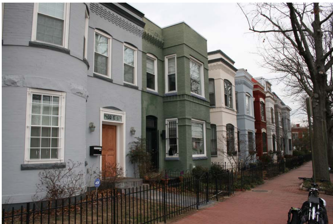
View of 1402 E Street SE looking northeast
