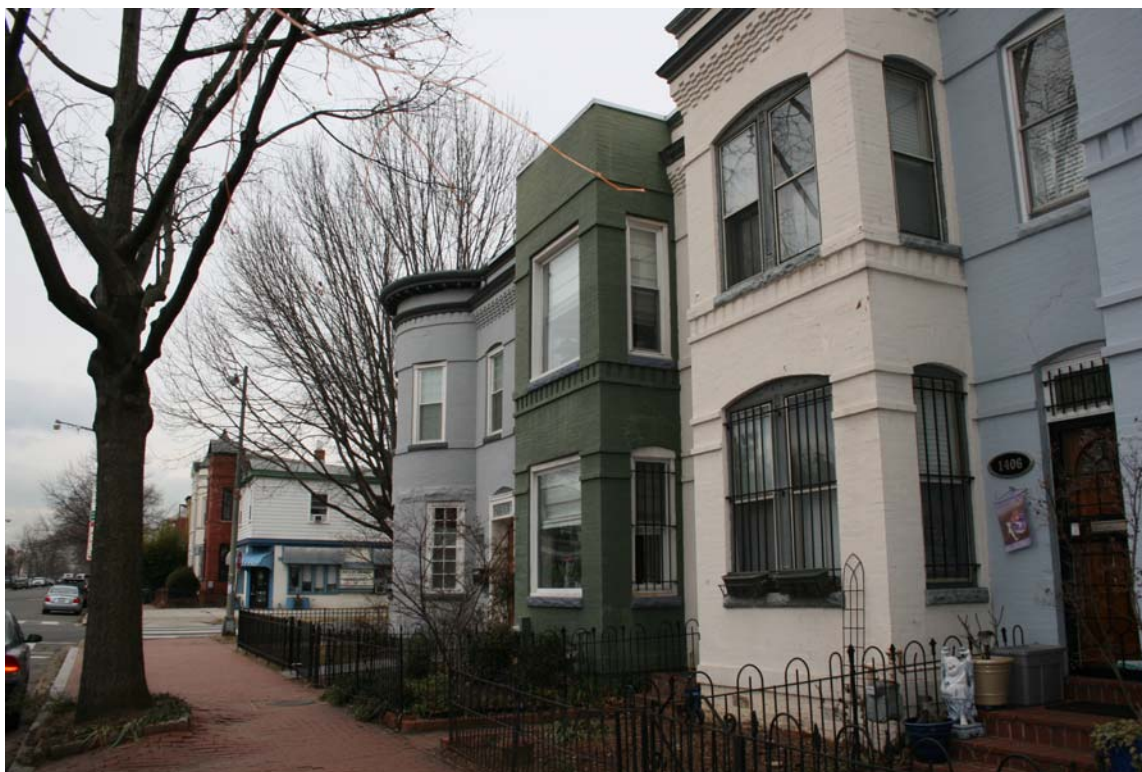
View of 1402 E Street SE looking northwest
