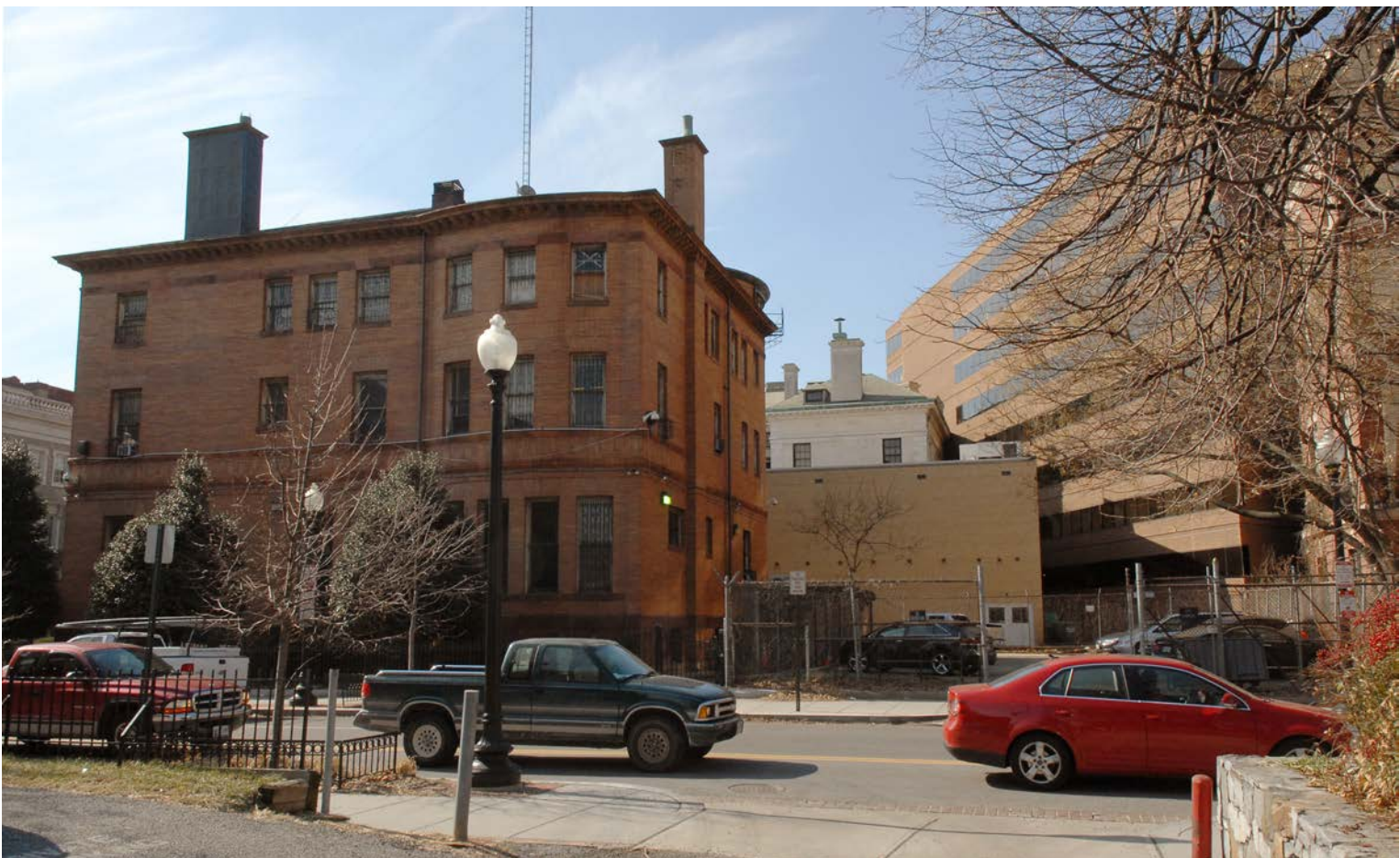
View from 18th Street
