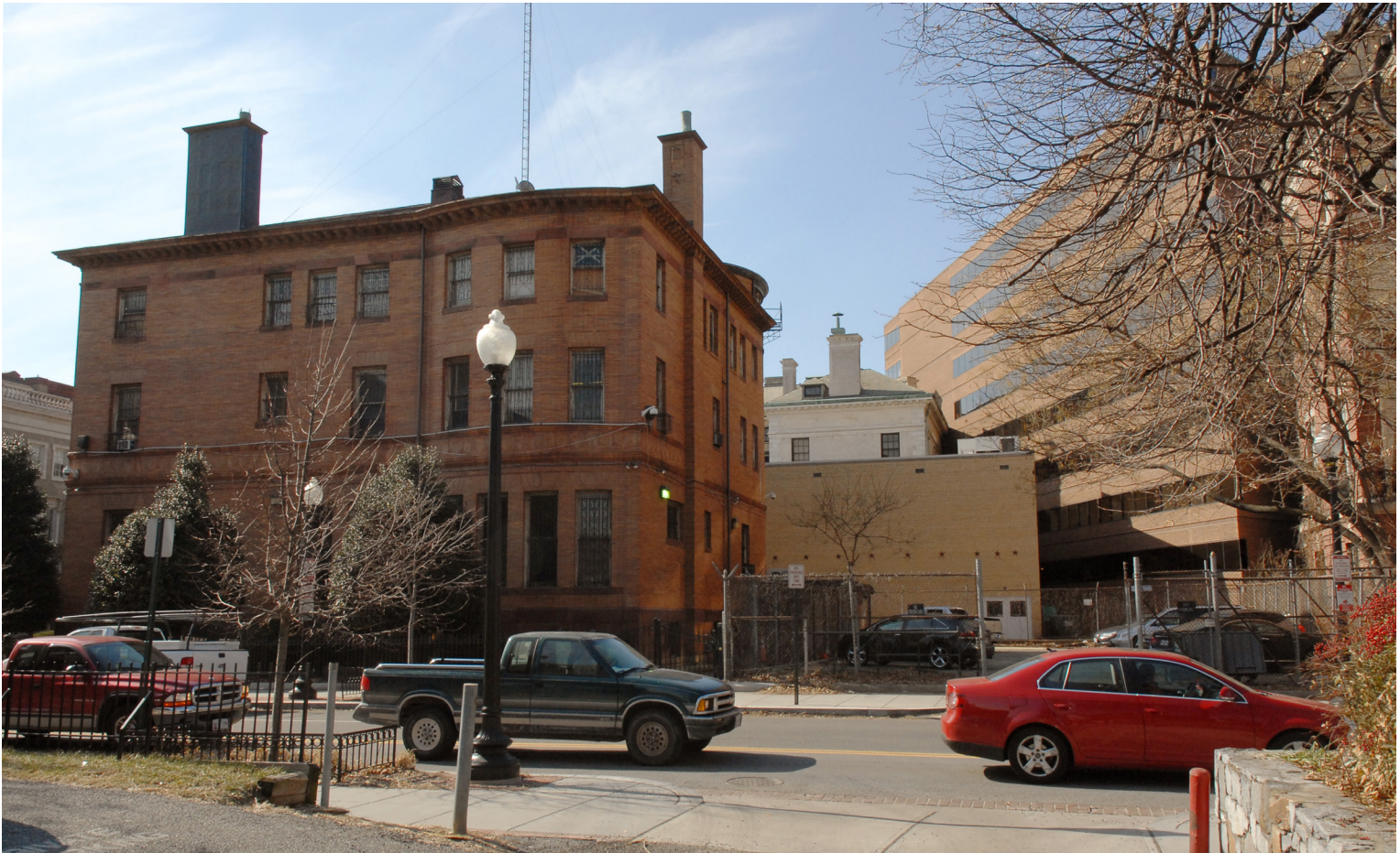
View from 18th Street
