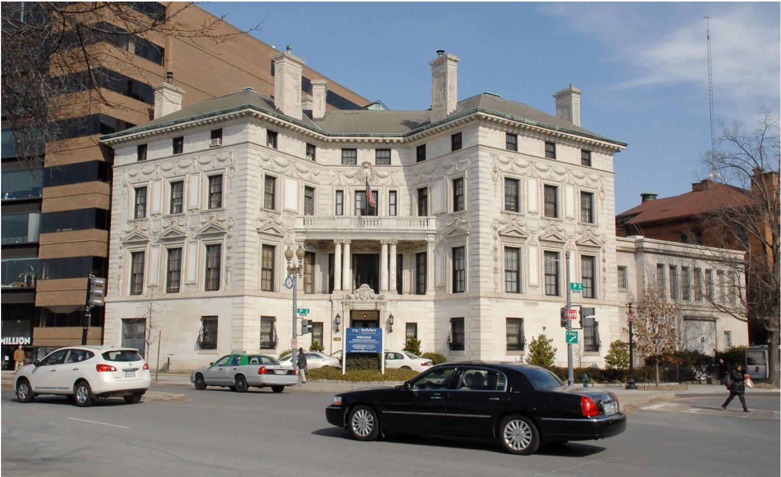
View from Dupont Circle
