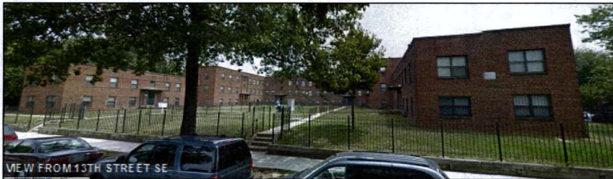
BUILDING 1 – 3232-3242 13 th Street SE
