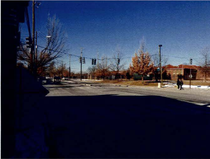
Figure 8: Pavement Conditions - 13 th Street and Alabama Avenue (looking west)
