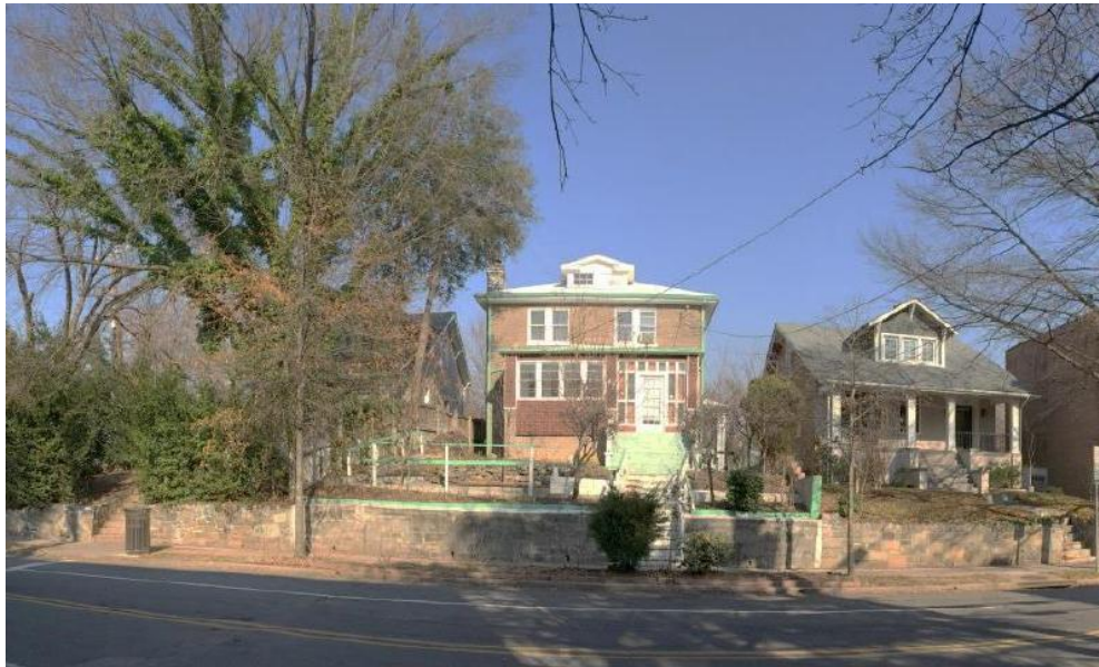
Subject Property (current structure to be demolished)
