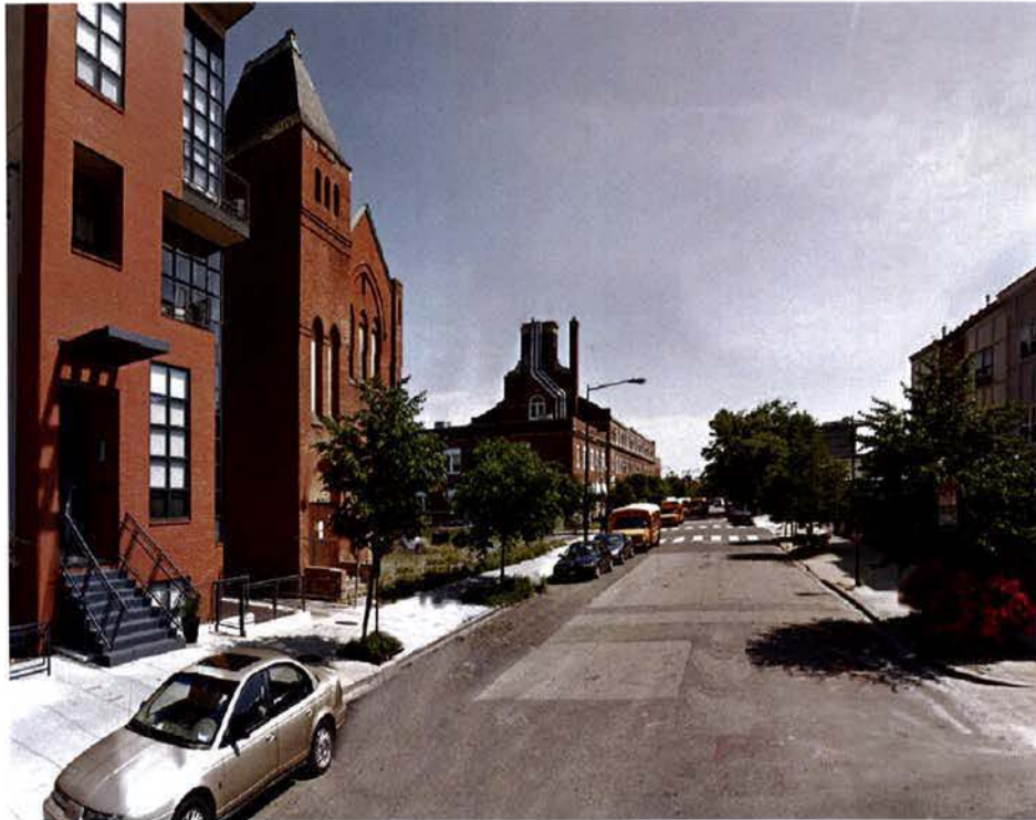
VIEW FROM 10TH STREET
