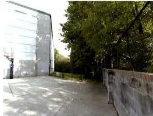
IMAGE D: SOUTHWEST CORNER
