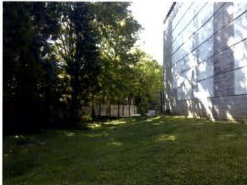
IMAGE B: SOUTH ELEVATION LOOKING WEST
