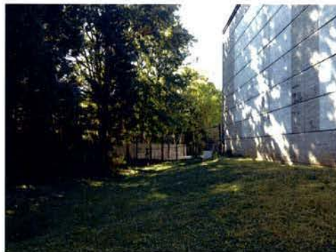
IMAGE B: SOUTH ELEVATION LOOKING WEST
