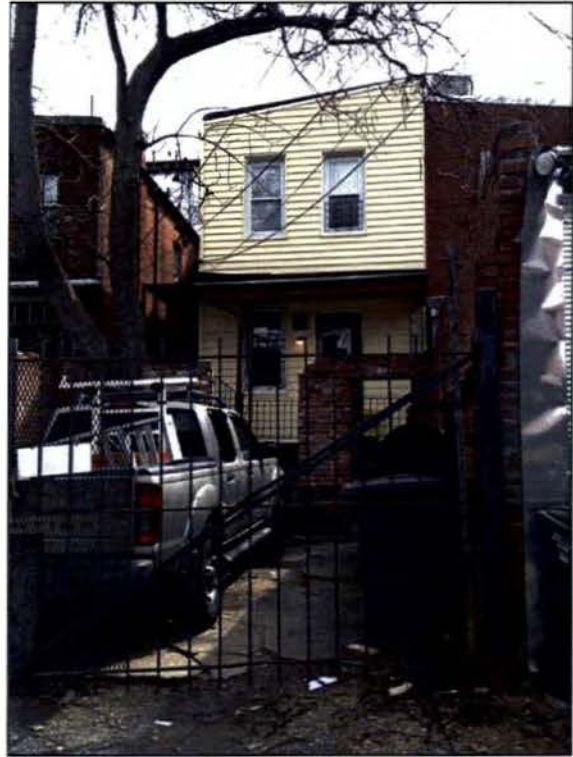
REAR OF PROPERTY FROM REAR ALLEY
