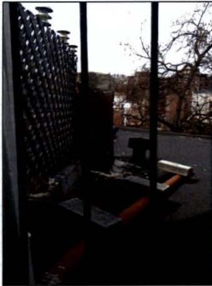
ROOF ON THIRD LEVEL
