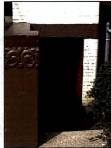
ENTRANCE TO LOWER LEVEL
