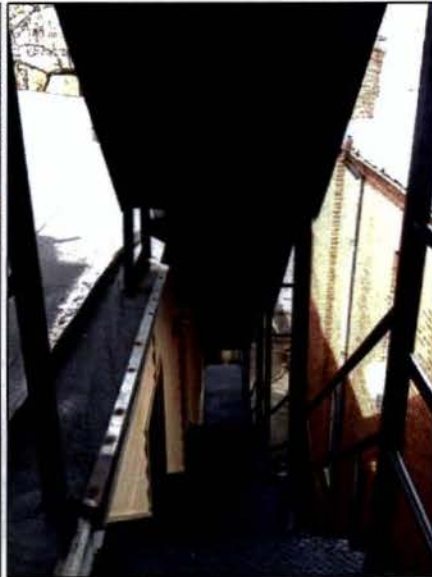
EXTERIOR FIRE STAIRS
