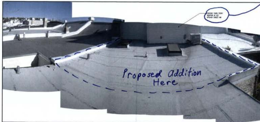
IMAGE OF EXISTING ROOF
