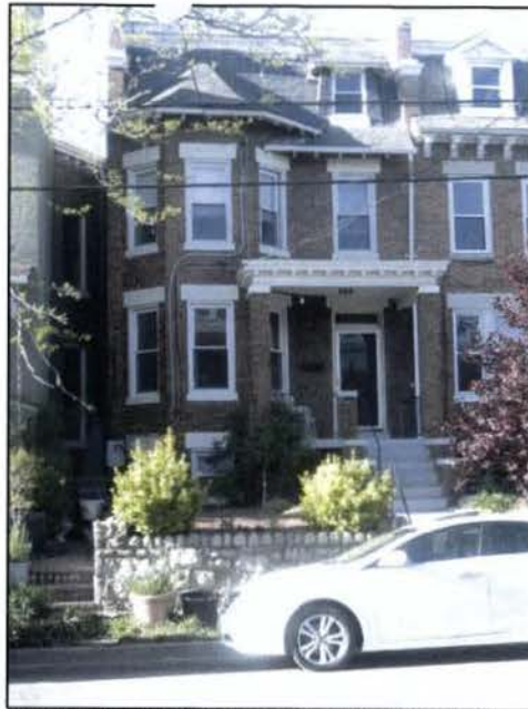
IMAGE OF FRONT OF HOUSE (SOUTH ELEVATION)
