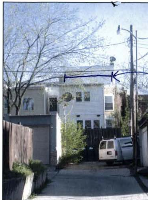
IMAGE OF BACK OF HOUSE (NORTH ELEVATION)
