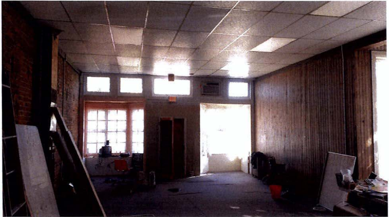
Interior of the "Commercial Space" in the Building
