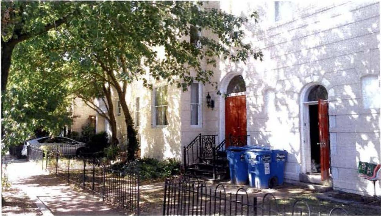
View of 2 Entrances Along 13 th Street, Including the Residential Entrance
