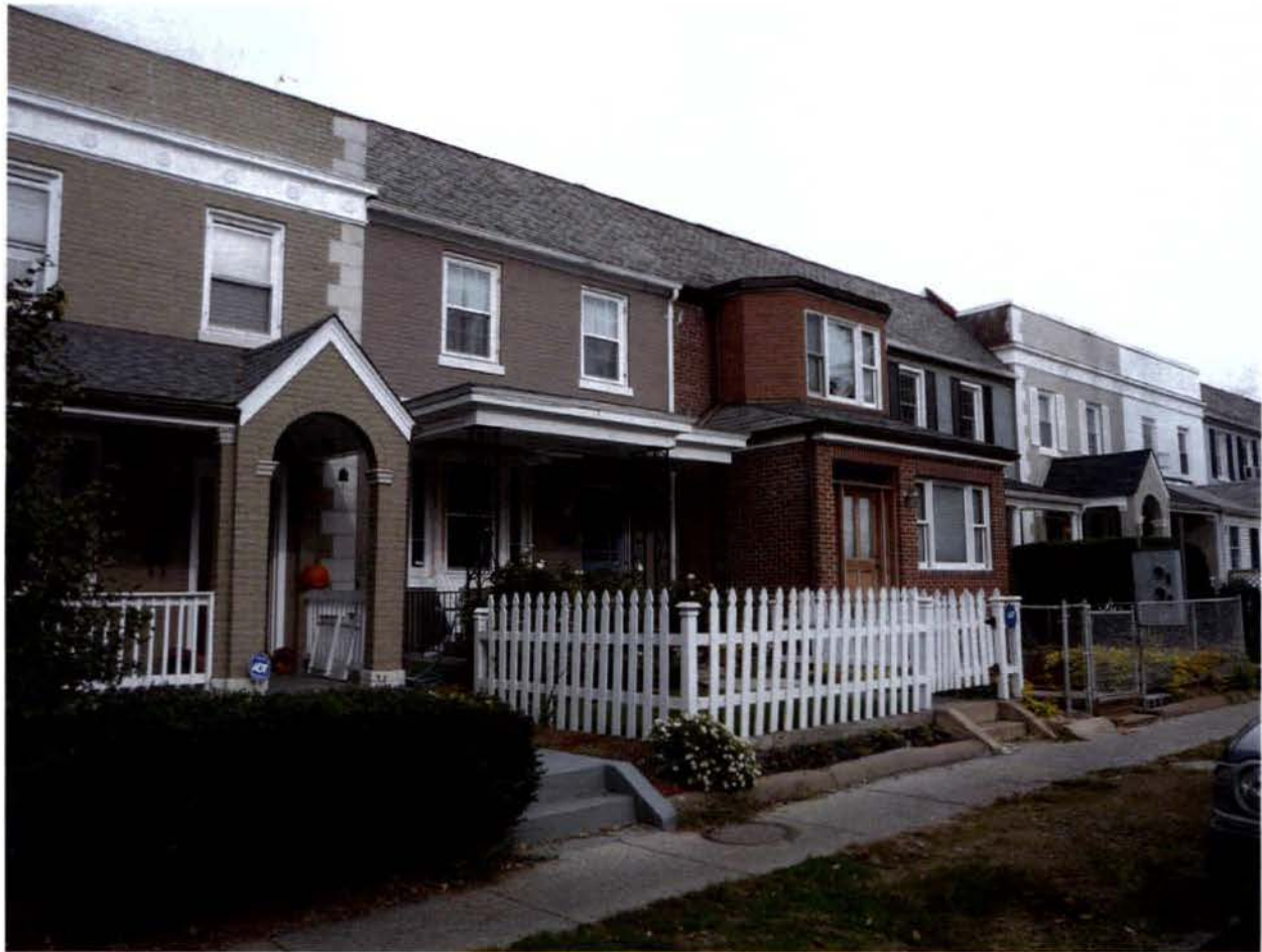
S) 1433 2-Story Addition & Porches - (south side of 1400 block)
