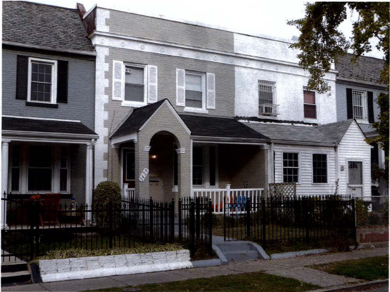
R) 1427 Enclosed porch - (south side of 1400 block)
