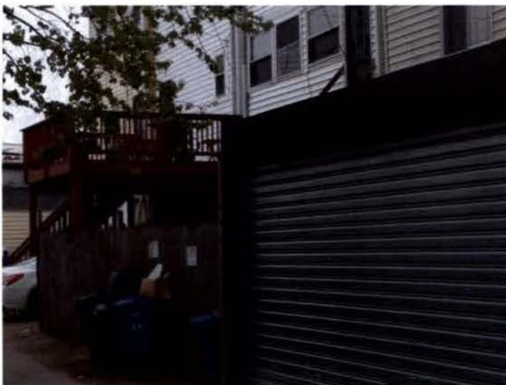
I) 1400 Parkwood Place additional decks in existence - (facing east)
