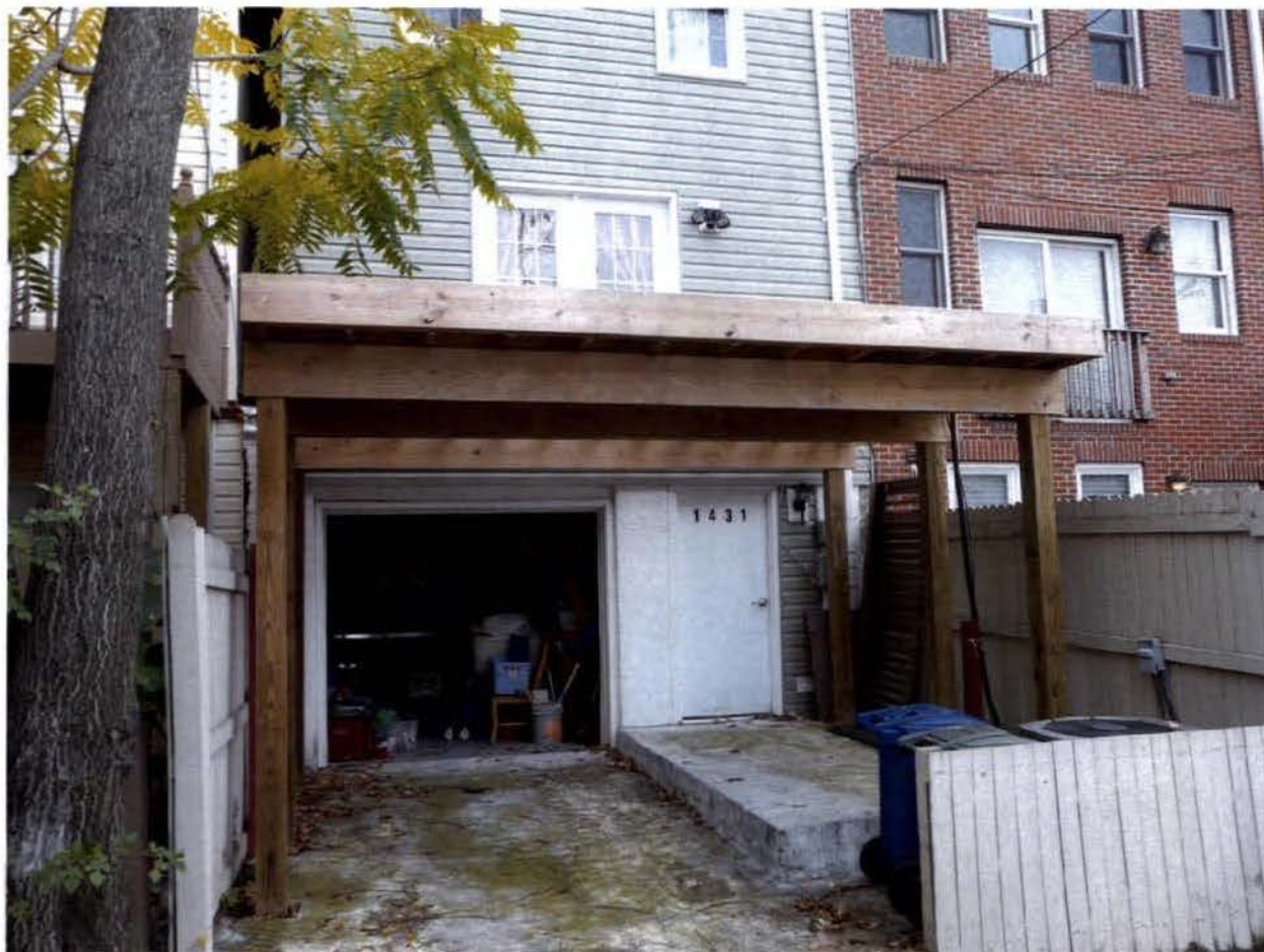
A) 1431 Parkwood Place NW – (rear elevation)
