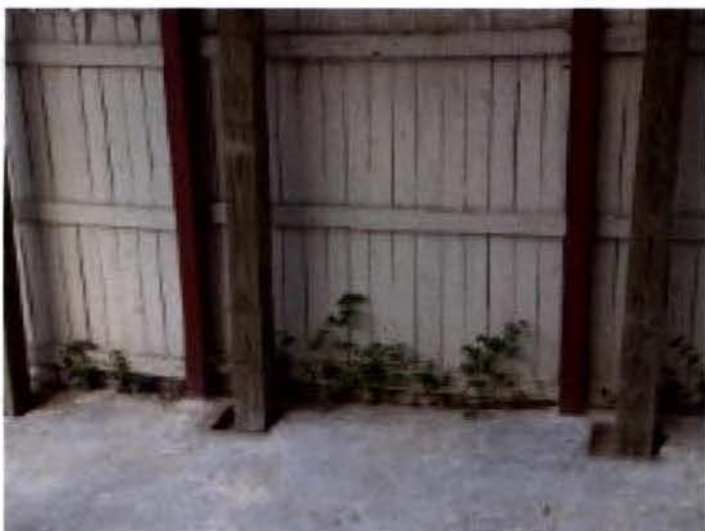
B) 1431 Parkwood Place existing deck posts - (old and new)
