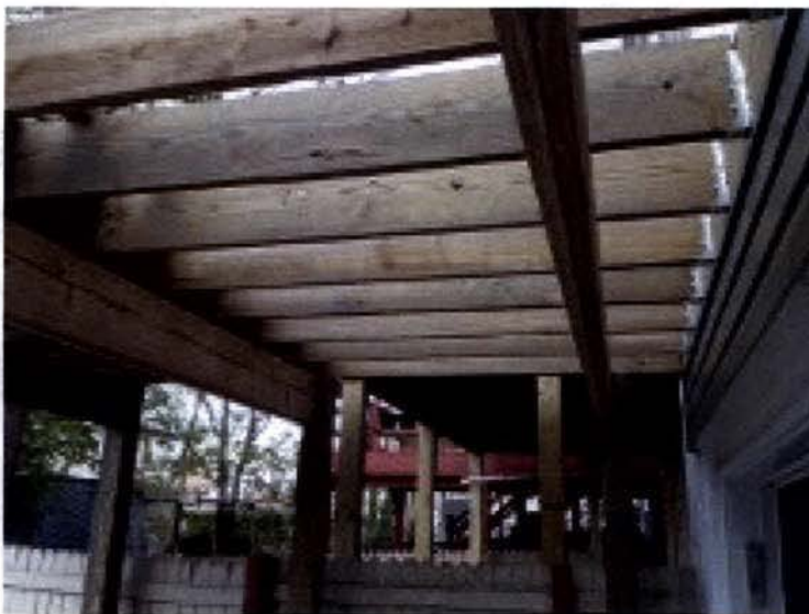
F) 1431 Parkwood Place structure - (facing east)
