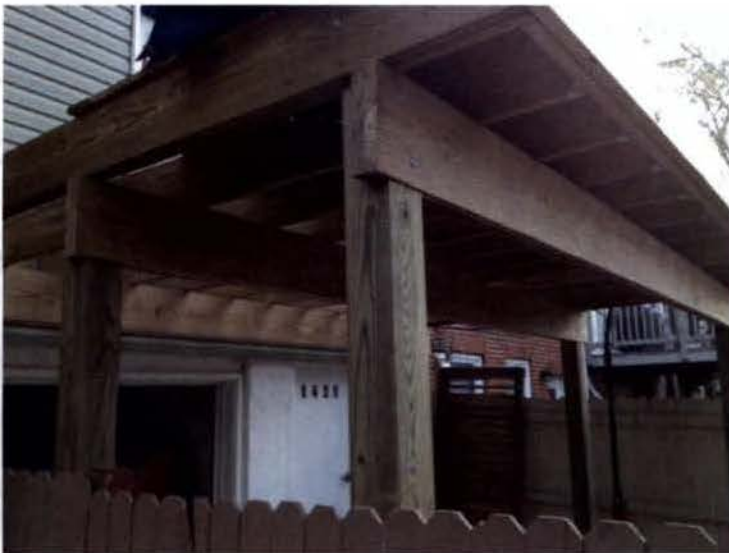
D) 1431 Parkwood Place existing structure - (facing west)
