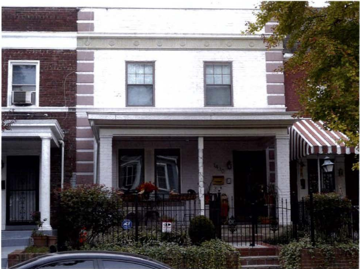
N) 1430 Parkwood Place - (north side wider lot space)
