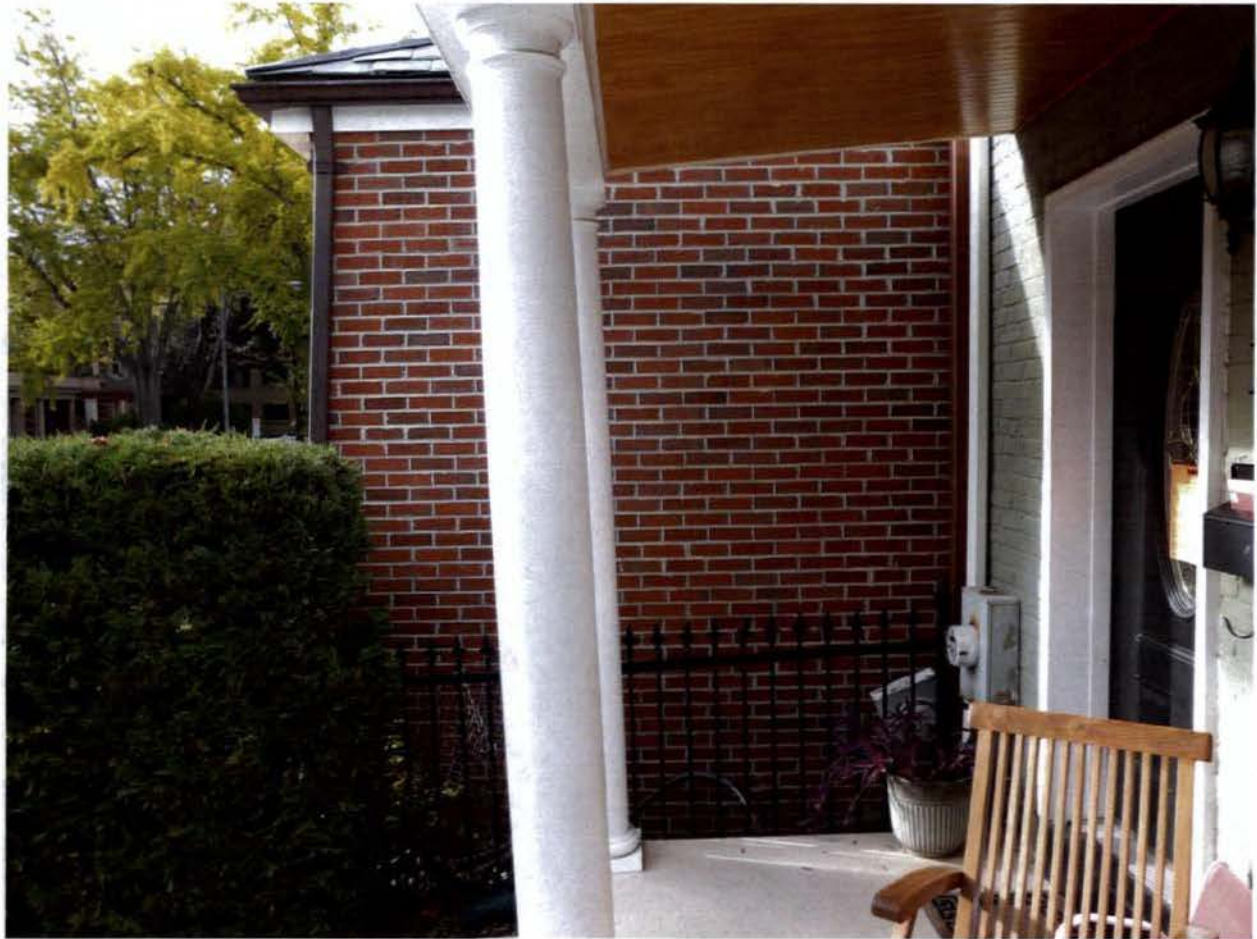
O) 1433 Parkwood Place 2-story addition wall - (from 1431 Parkwood Place south side)
