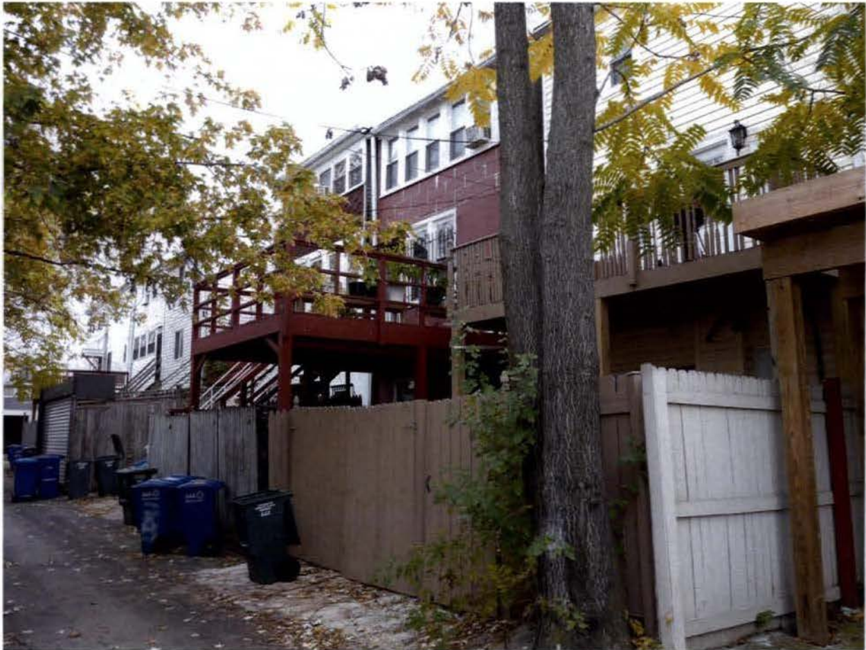
H) 1400 Parkwood Place block existing decks (facing south-east)
