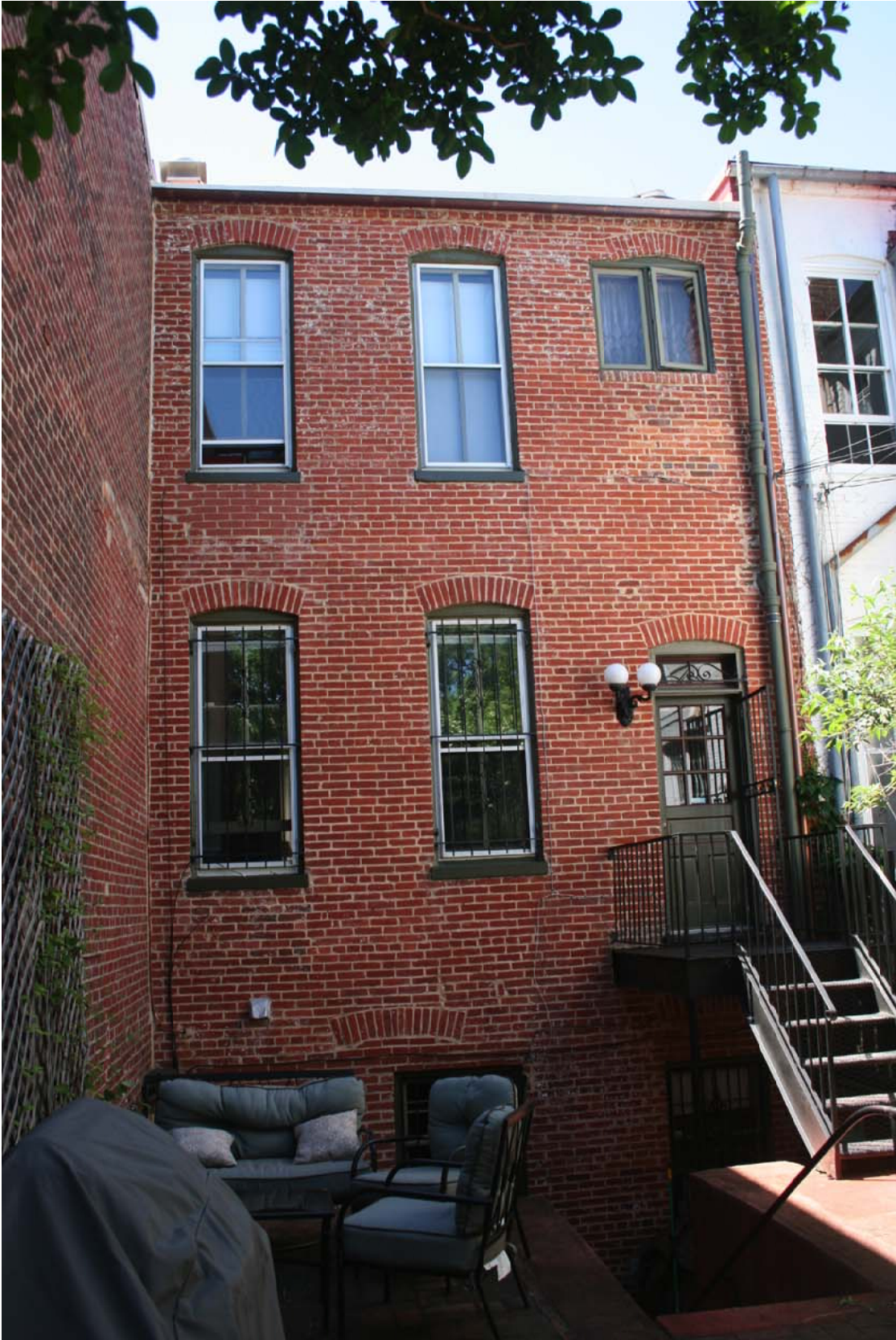
2 REAR OF HOUSE FROM YARD C-4
