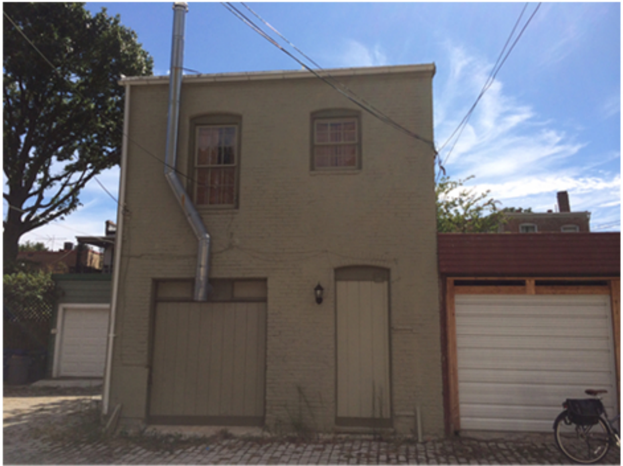
REAR VIEW OF PROPERTY/CARRIAGE HOUSE
