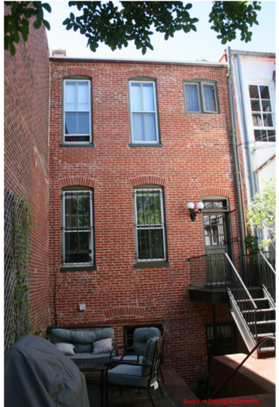
REAR OF HOUSE, FROM YARD
