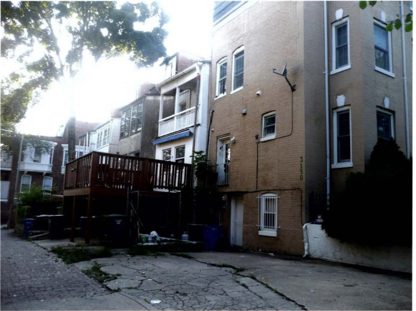
View from adjacent alley near 17th Street NW sidewalk. Proposed deck will be essentially same size as deck serving adjoining house.
