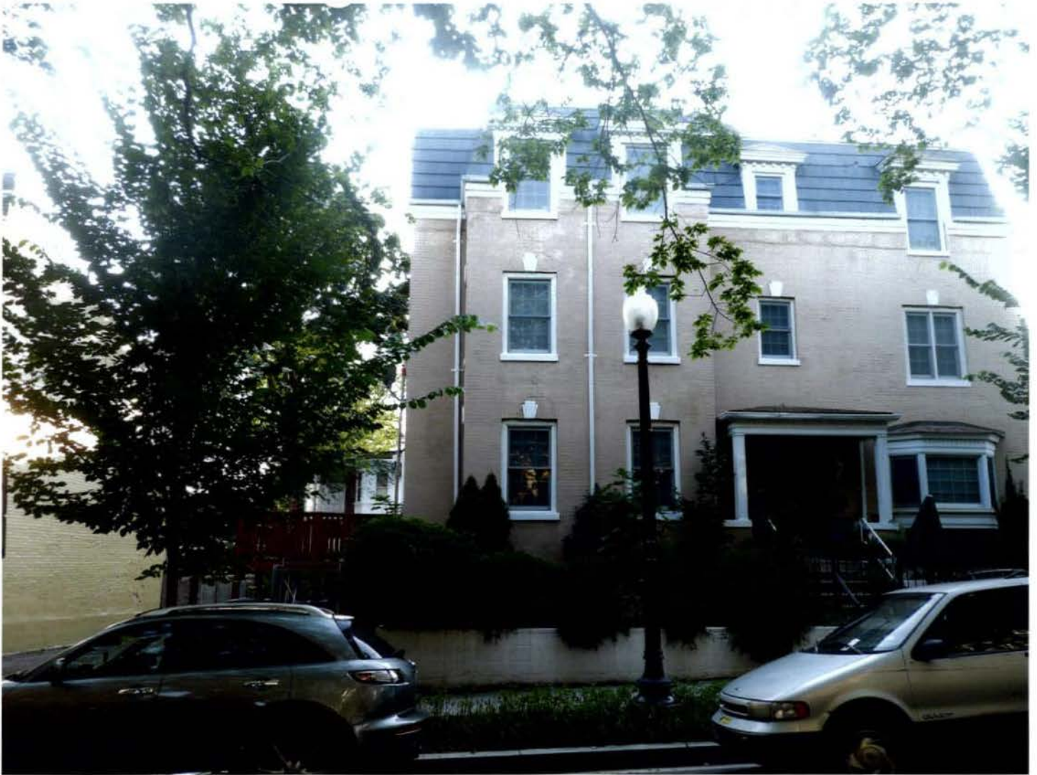
Front of house as viewed from across 17th Street NW. Dark red deck seen at left serves adjoining house.
