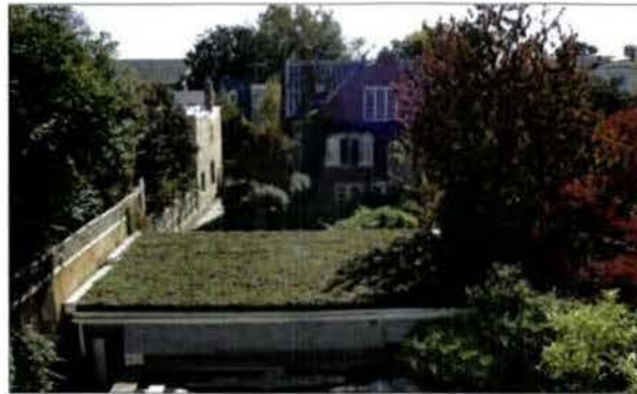
GREEN ROOF EXAMPLE
