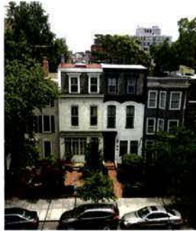
1617 19TH STREET, NW 1619 19TH STREET, NW
