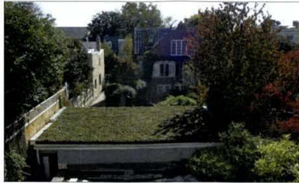
GREEN ROOF EXAMPLE
