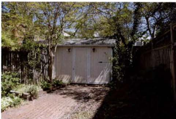
PHOTO #5: EXISTING ACCESSORY STRUCTURE AT REAR PROPERTY LINE. EXISTING REAR ACCESSORY STRUCTURE, TO BE REMOVED.
