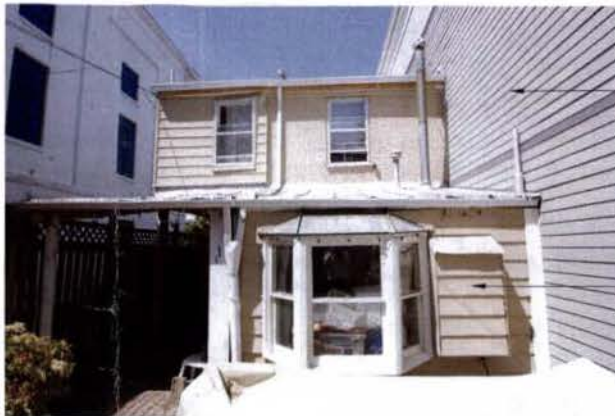
PHOTO #4: 508 4TH ST. SE, REAR FACADE. VIEW FROM REAR YARD. ADJACENT RESIDENCE TO NORTH, 506 4TH STREET, SE 508 4TH STREET, SE (EXISTING REAR ADDITION W/ ALUMINUM SIDING)
