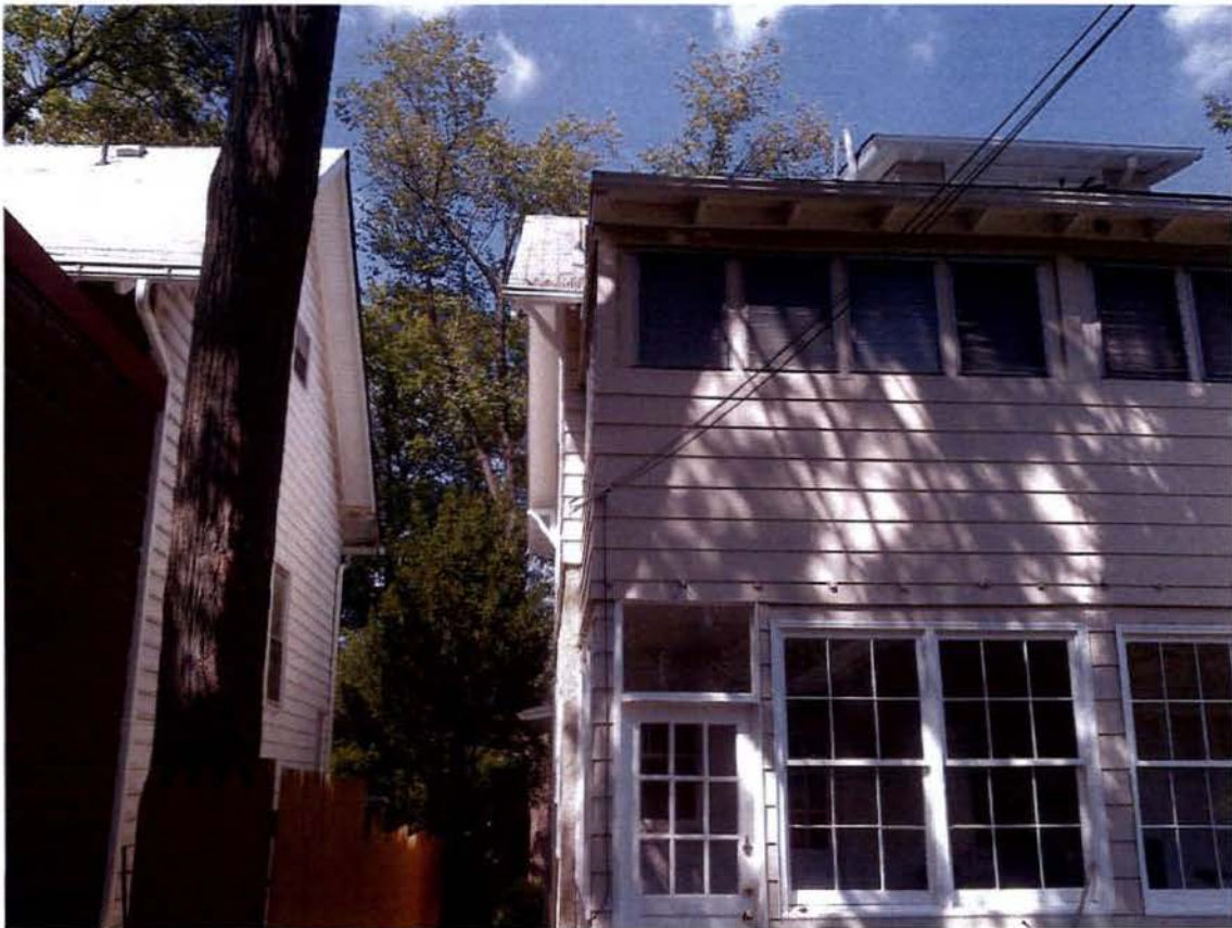
View of the Rear of 3704 and the Property to the West
