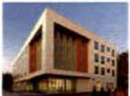
Brookland Artspace Lofts
