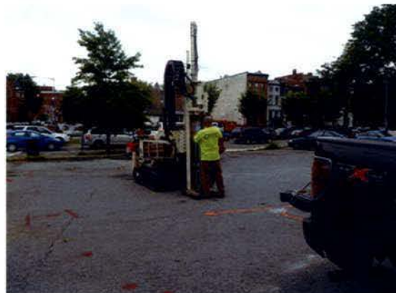
View of SB 9 being advanced.
