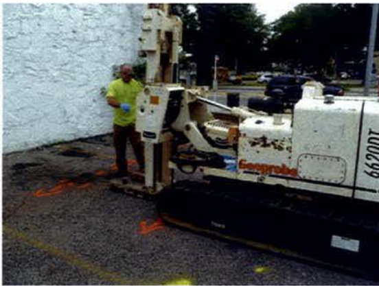
View of test boring SB3 being advanced.
