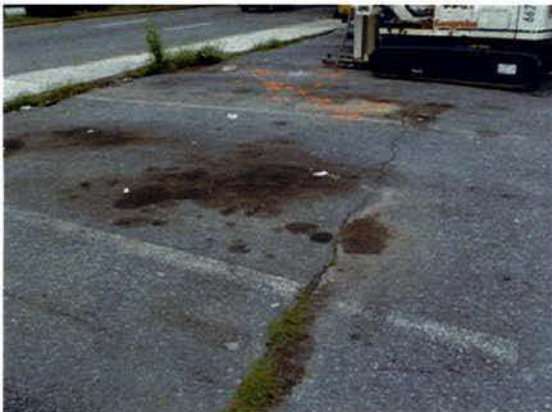
View of asphalt patch over old tank locations.
