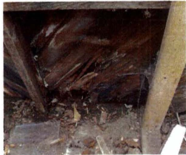
East Wall - existing condition
