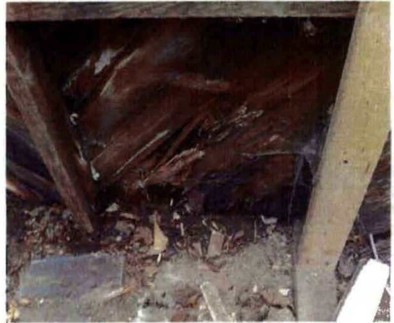
East Wall - existing condition
