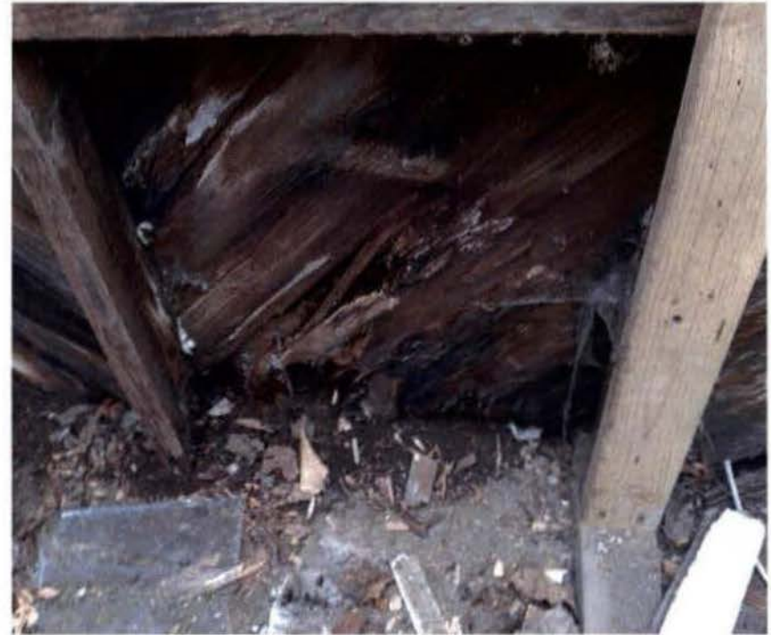
East Wall - existing condition
