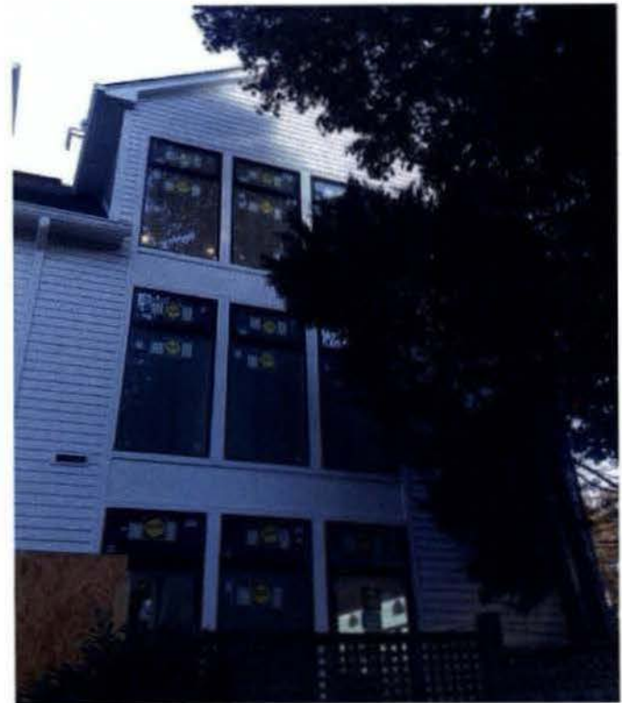
Construction West Elevation
