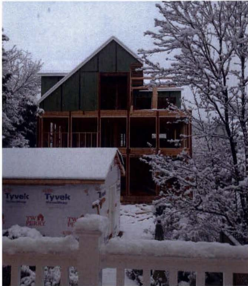
Early winter construction - 2013
