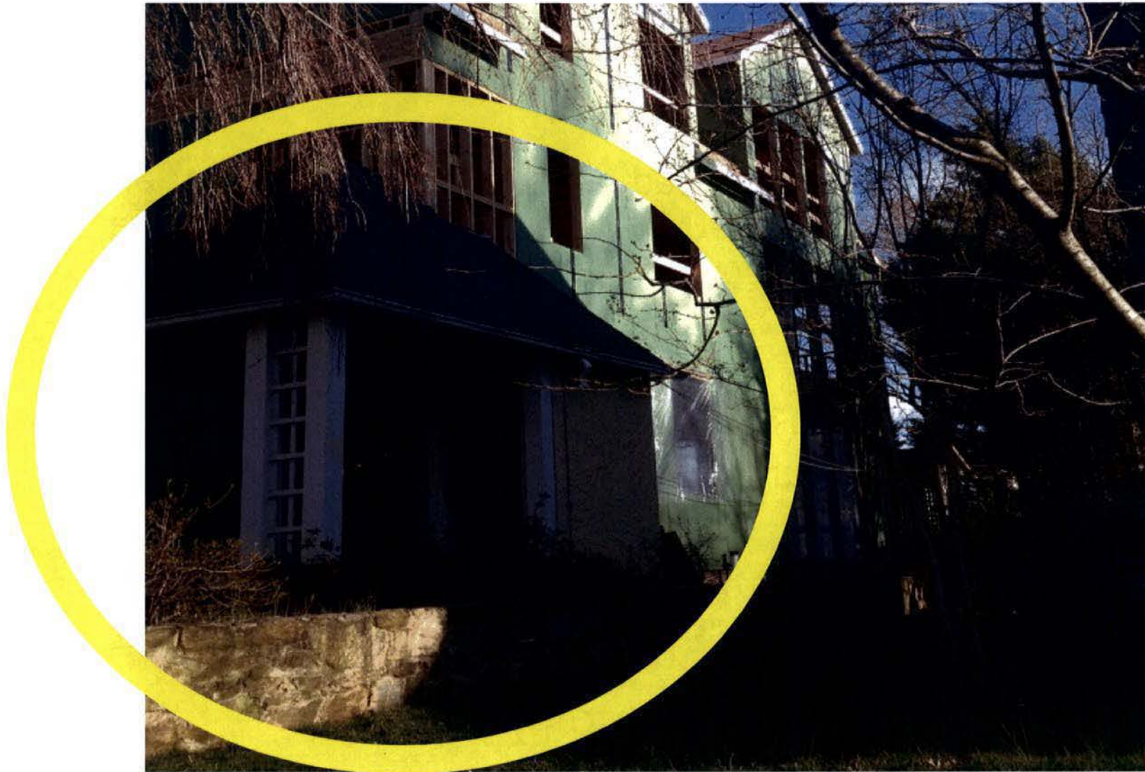
Photo Showing area of existing porch to be removed
