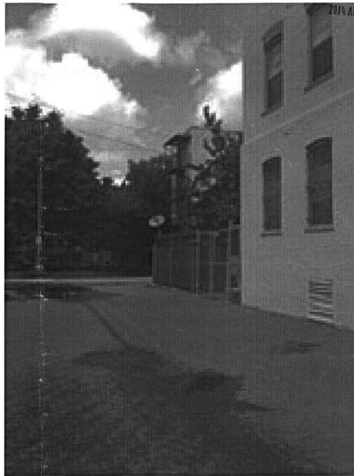
2 C-6 VIEW FROM ALLEY, LOOKING NORTH
