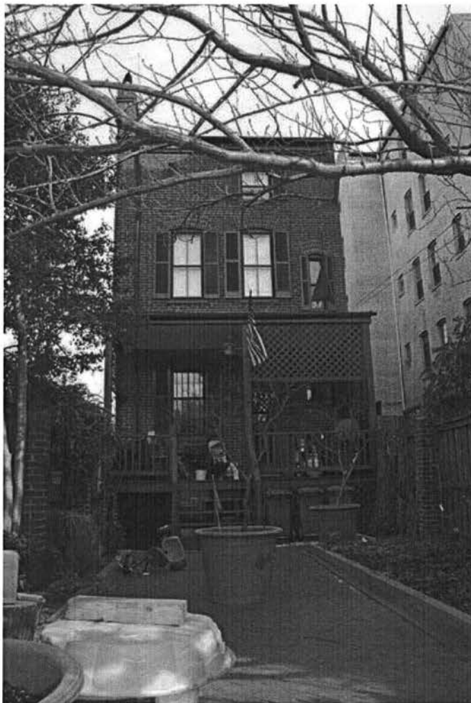
1 REAR OF HOUSE C-4
