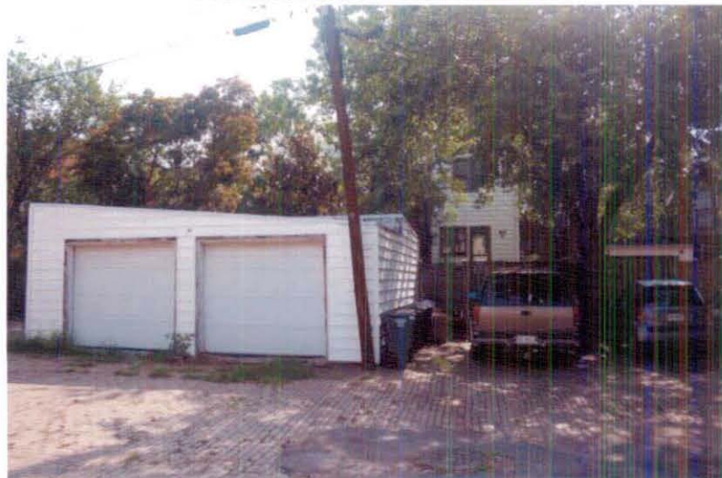
Alley View of 761 10 th Street SE
