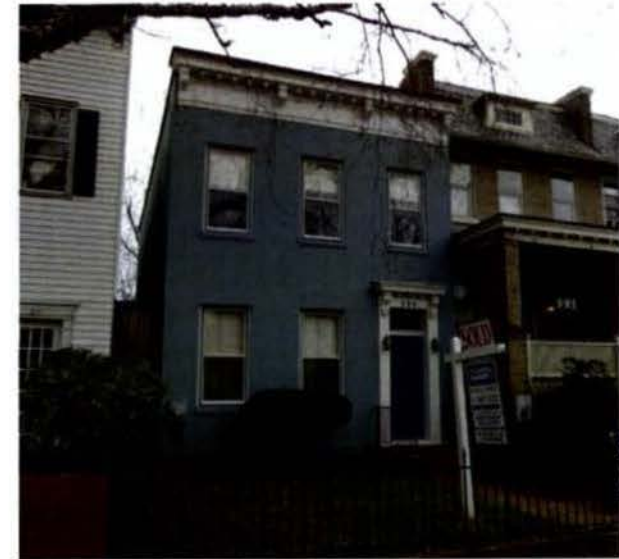
PHOTO: FRONT FACADE
