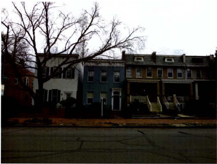
PHOTO FRONT: EAST ELEVATION
