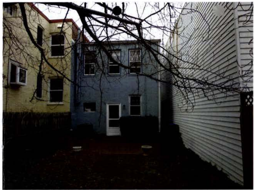
PHOTO REAR: WEST ELEVATION
