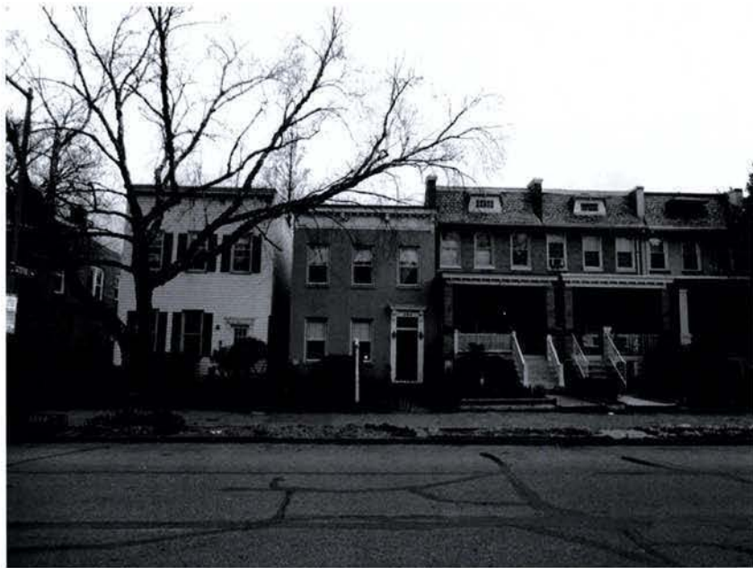
PHOTO FRONT: EAST ELEVATION
