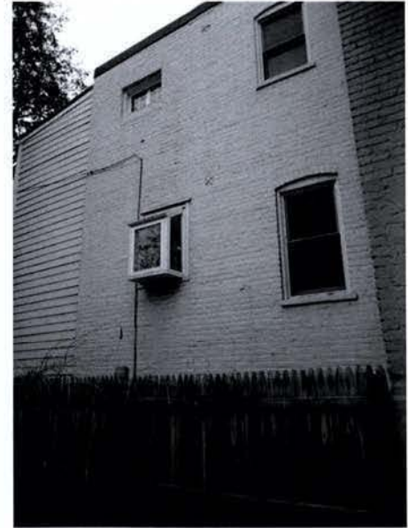
PHOTO REAR: FACING NORTH
