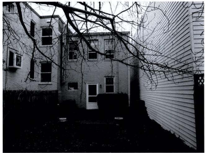
PHOTO REAR: WEST ELEVATION
