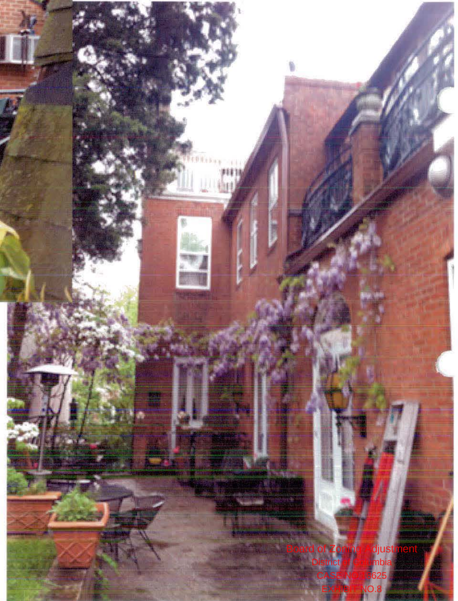
REAR OF HOUSE, EAST SIDE
