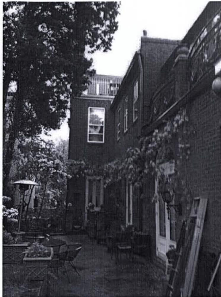
2 REAR OF HOUSE, EAST SIDE C-5
