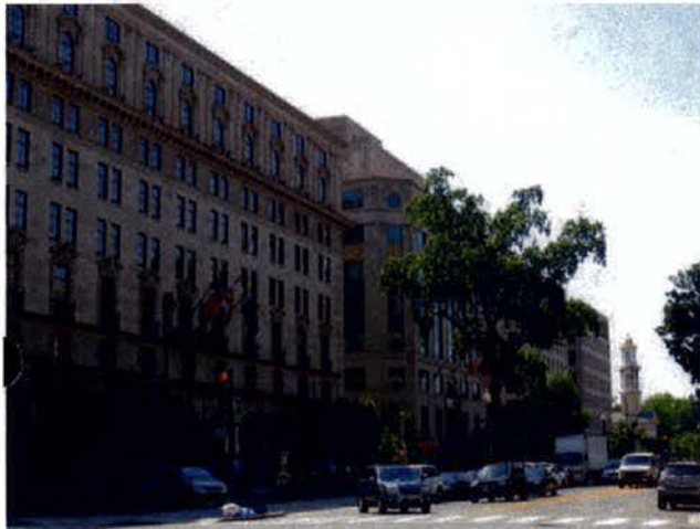
4) VIEW FROM 16TH STREET NW LOOKING SOUTH
