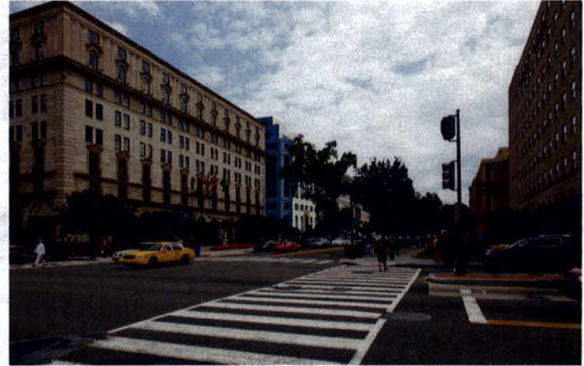
2) VIEW FROM 16TH STREET NW LOOKING SOUTH
