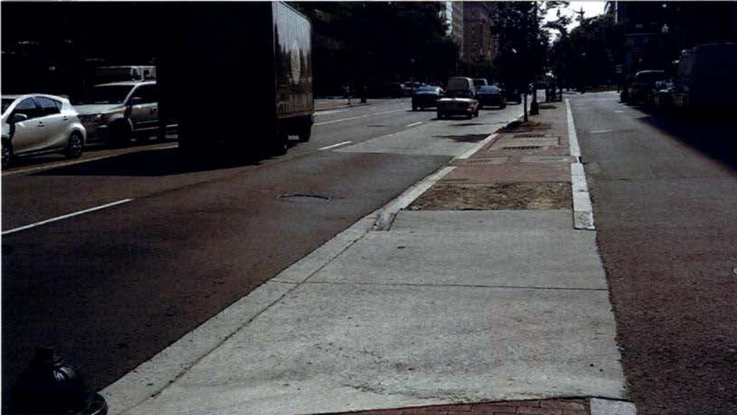
Right Turn Egress to EB K Street Mainline Continued (taken 8/9/2013)
