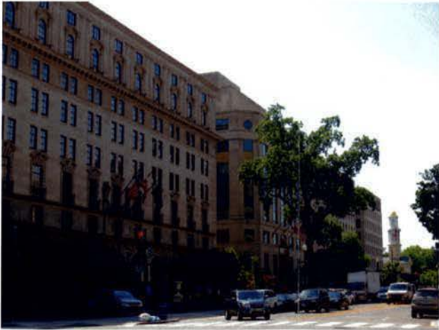
4) VIEW FROM 16TH STREET NW LOOKING SOUTH
