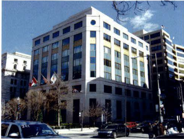
1) VIEW FROM 16TH AND EYE STREET NW LOOKING NORTH-EAST
