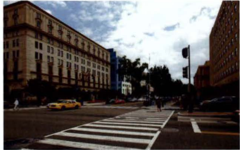
2) VIEW FROM 16TH STREET NW LOOKING SOUTH
