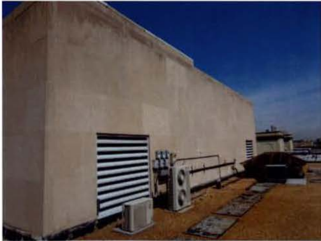
4) VIEW OF LOWER PENTHOUSE EAST ELEVATION
