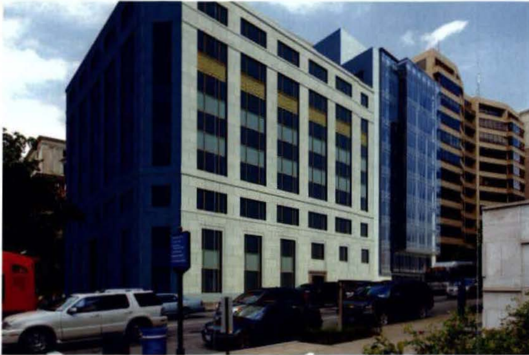
VIEW FROM 16TH AND EYE STREET NW LOOKING NORTH-EAST
