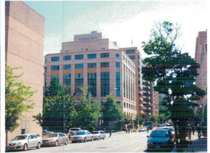
3) VIEW FROM EYE STREET NW LOOKING EAST
