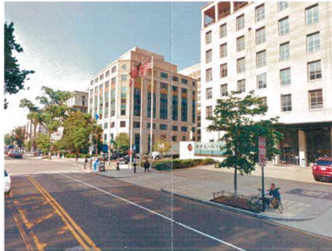
5) VIEW FROM 16TH STREET NW LOOKING NORTH
