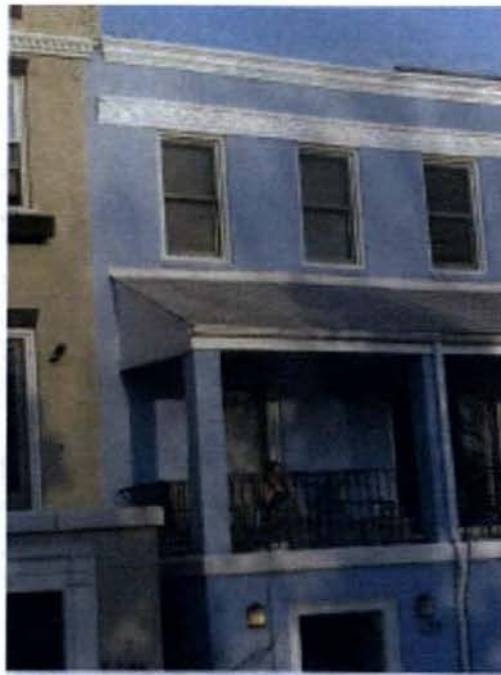
PARTIAL WEST FACADE
