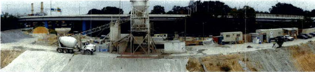
VIEW OF I-395 @ ±55' (GROCERY PARKING P1)
