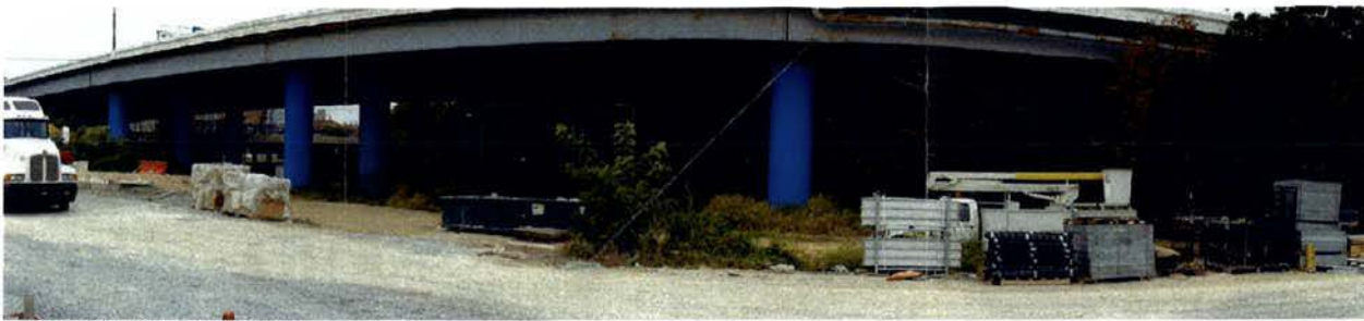
VIEW OF I-395 @ ±32' (GROCERY LEVEL)
