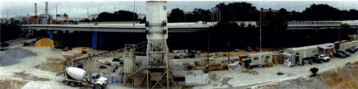
VIEW OF I-395 @ ±67' (GROCERY PARKING P2)
