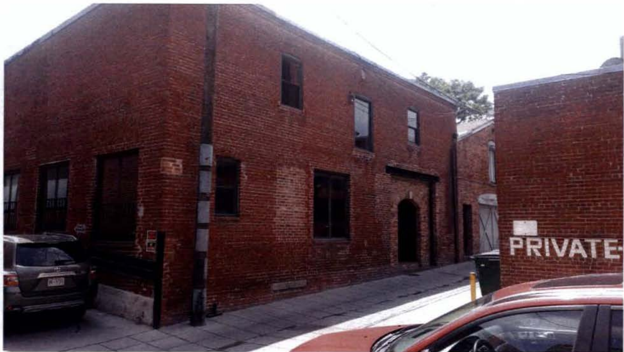
View of the vacant building ("Building A") from across the alley
