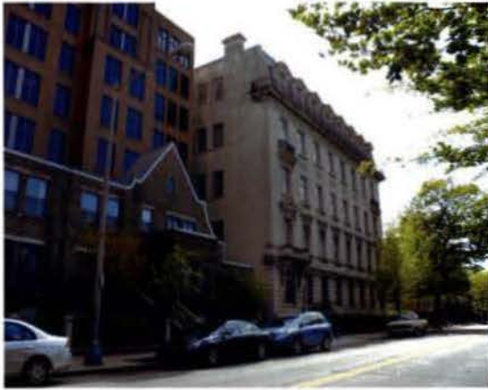
1 - View from P Street Looking West
