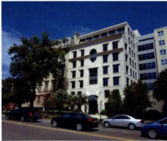
3 - View from Massachusetts Ave.
