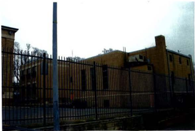
PHOTO - LEFT SIDE/REAR - FROM ALLEY
