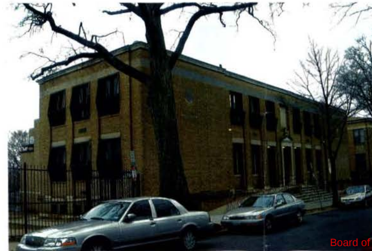
PHOTO - FRONT/LEFT END - FROM NEAL ST. N.E.
