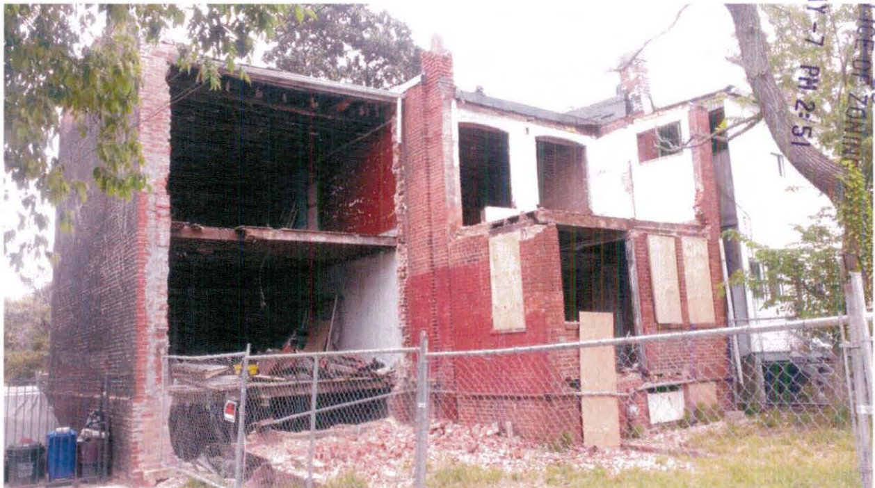
Rear Views of the Property after partial demolition
