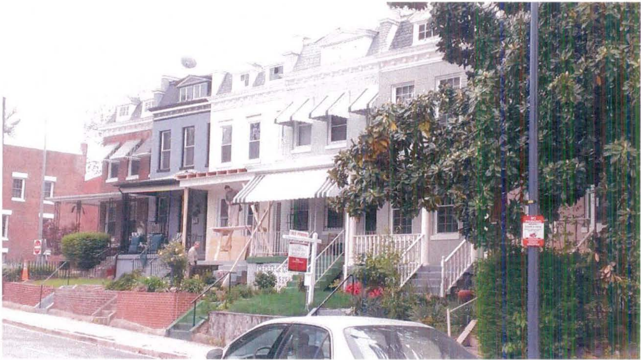
Buildings to the south of the Property
