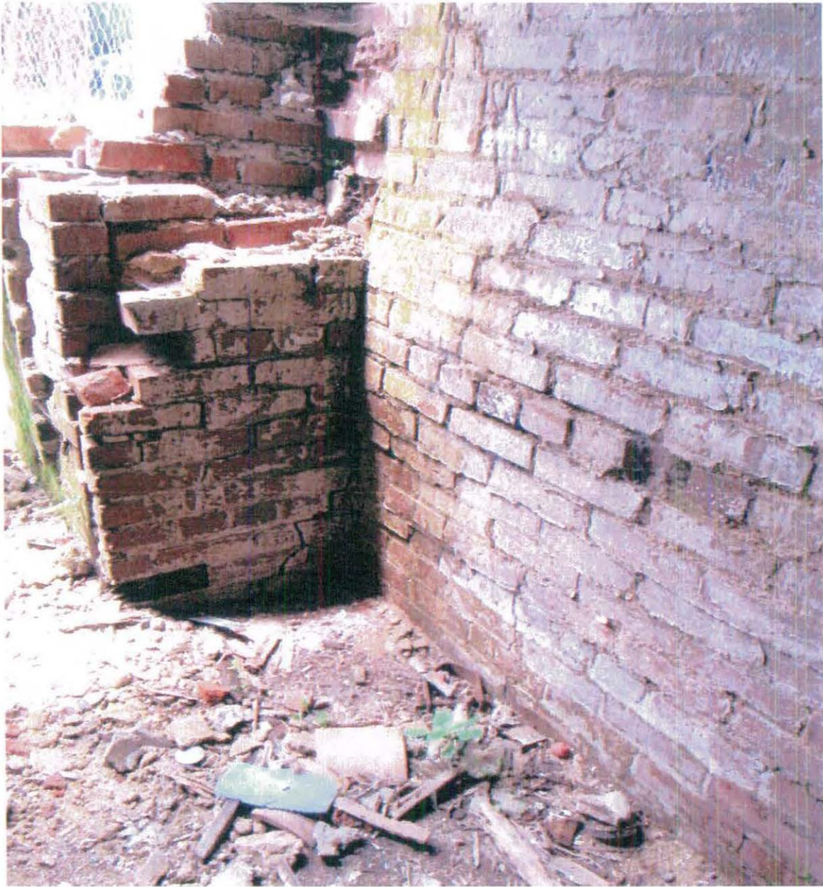
Hydrostatic Pressure on Masonry Walls
